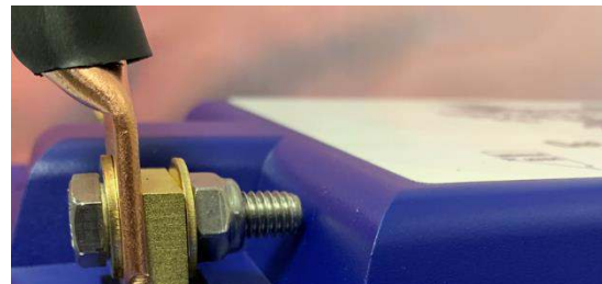
Improper Connection: One lug used with longer bolt creates interference with battery case
